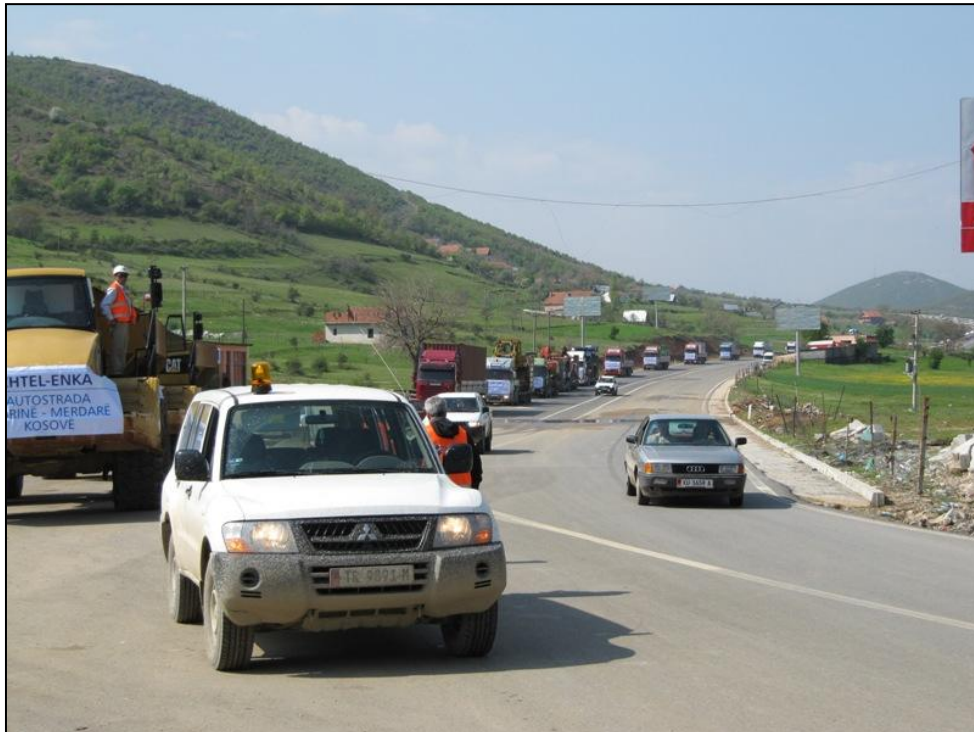
Photo 4 – Equipment Mobilization, 18 April
