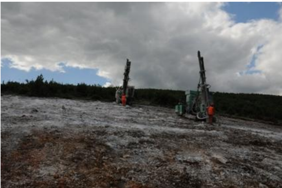
Photo 4 – Drilling for Blasting
