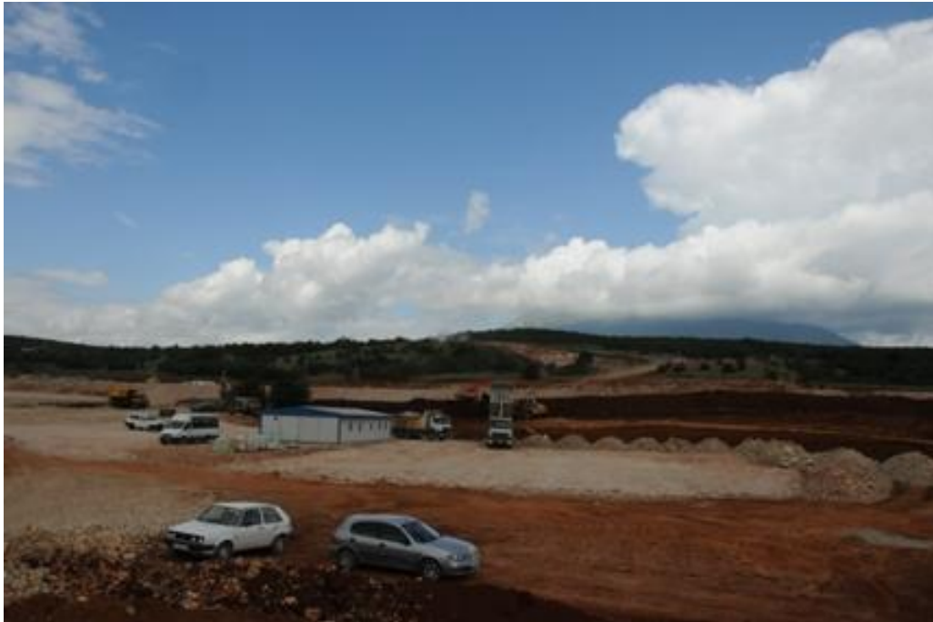
Photo 7 – Pre-Cast U Beam Plant Preparation
