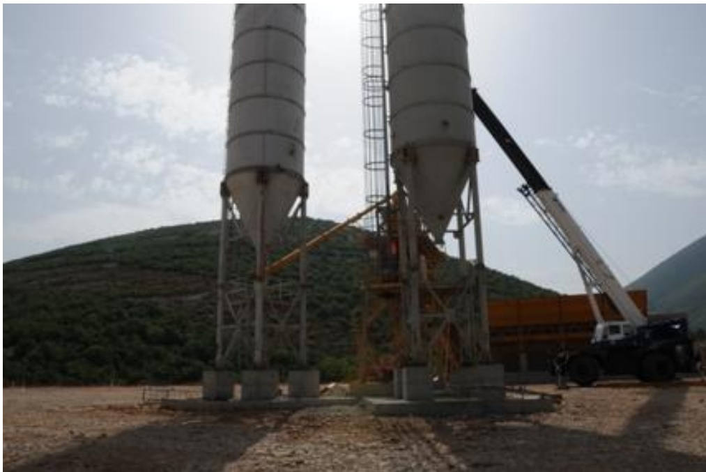
Photo 8 – Concrete Batch Plant Erection
