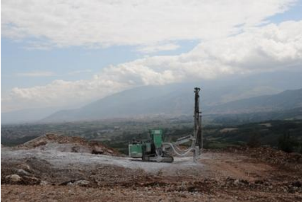
Photo 3 – Drilling for Blasting
